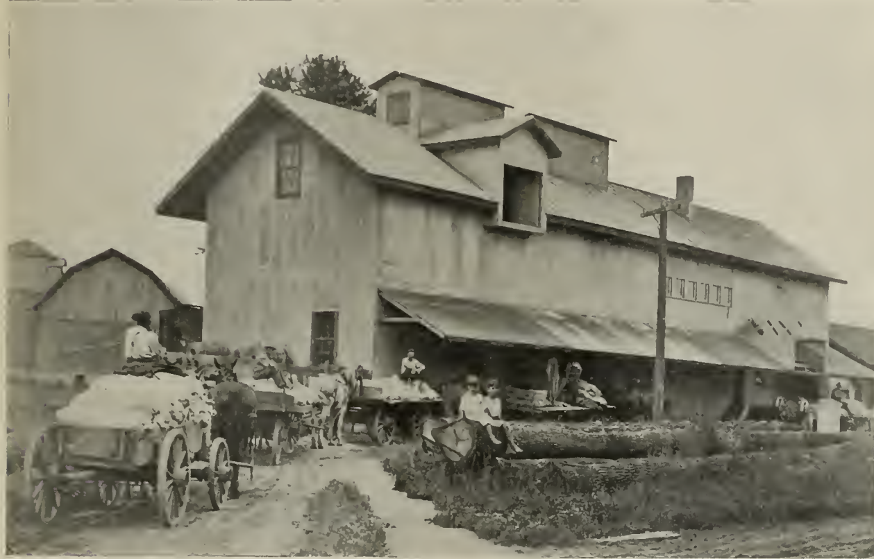
POST BROTHERS' ELEVATOR, ORLEANS, MICH.
